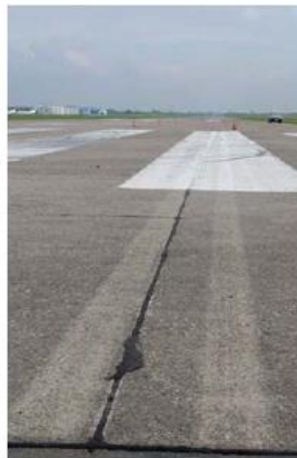
Above: figure - marks of hydroplaning on the runway
